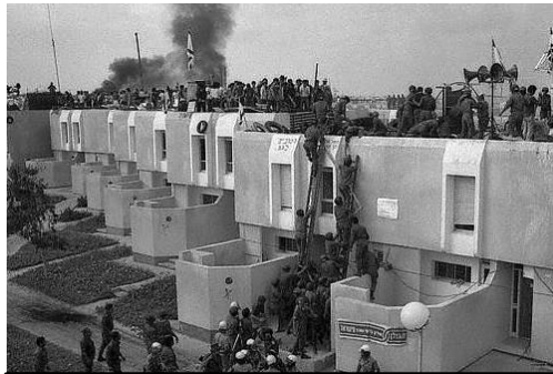
Yamit about to be demolished
