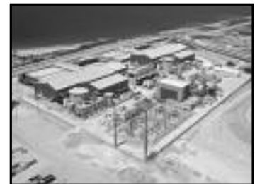
The Desalination Plant at Ashkelon
